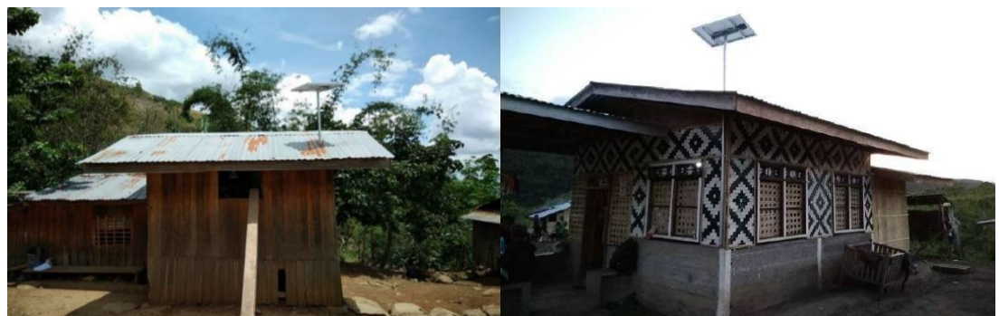
Diagram 7: Roof-through Pole mounted installations on GI roofs
