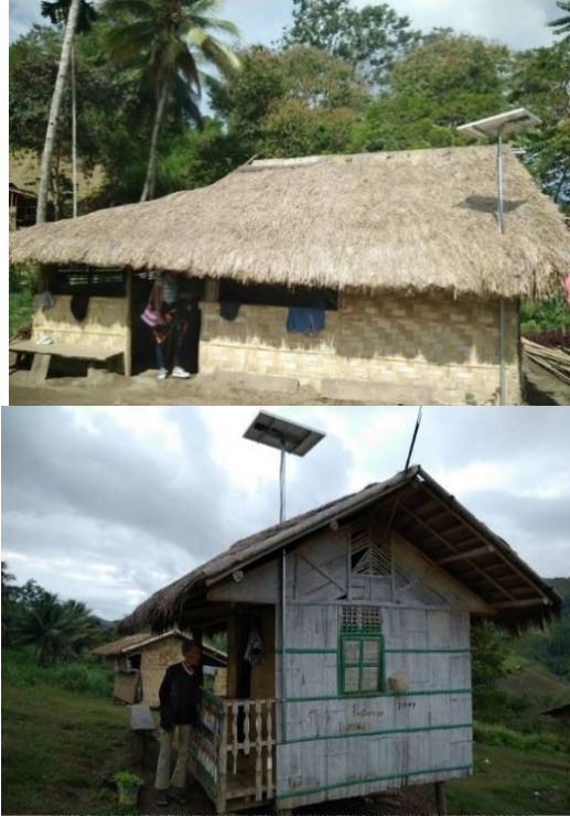
Diagram 8: Roof-through Pole mounted installations on thatched roof
